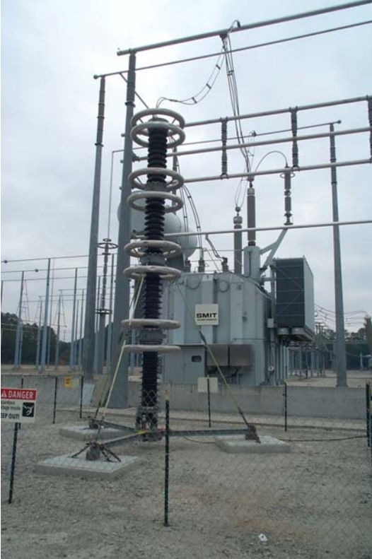
BPA Divider Installation @ GA Power Figure 1
